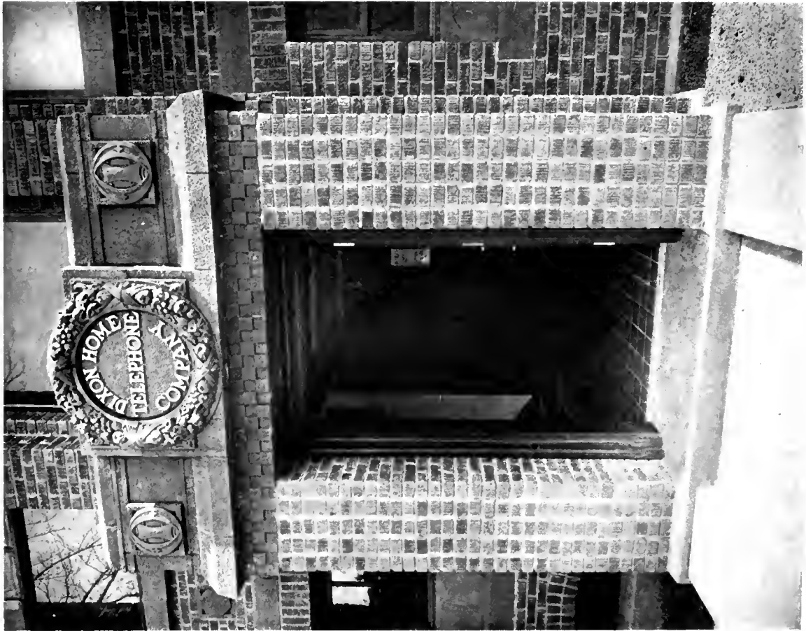
MAIN ENTRANCE DETAIL
